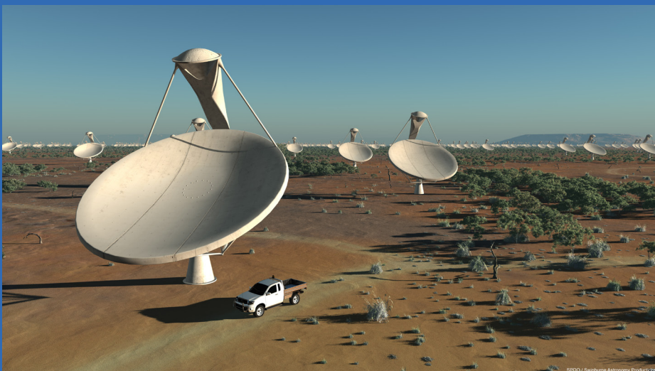
FIGURE 3: Artist's impression of the offset Gregorian antennas of the Square Kilometer Array, which will be built in South Africa and Australia.
